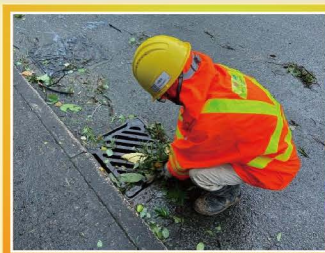
清理排水渠 Clearing of drainage channels
