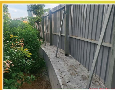
豎立圍板 Hoarding Erection
