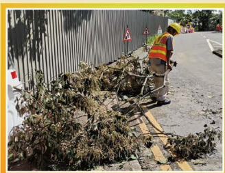
清理堵路的塌樹 Clearing of collapsed trees blocking the roads
